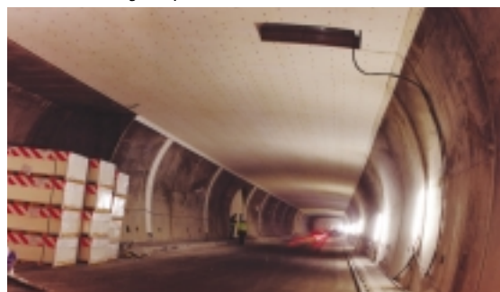
Figure 33 Toulon tunnel protected with the PROMATECT®-T boards for ceiling, escape routes, smoke extraction ducts and fire doors.
