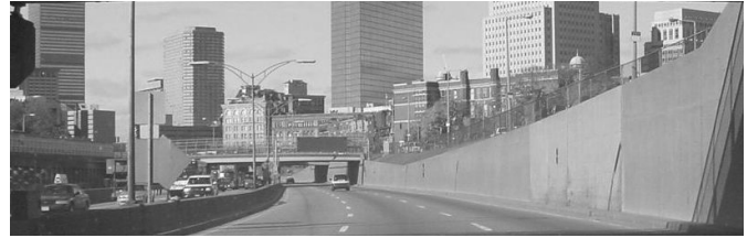
FIGURE A.3.3.32.1 Depressed Highway.
