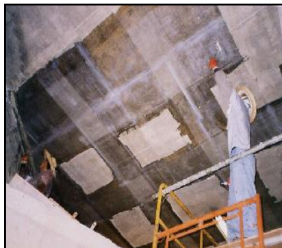
Adhesion of glass fiber
