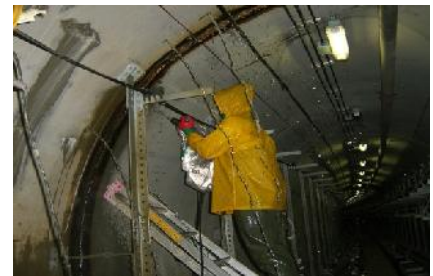
Hole drilling
