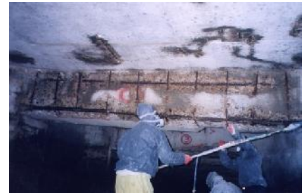
Removal corrosion in steel
