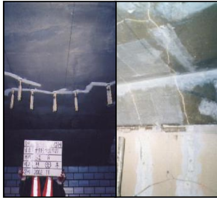
Crack sealing/ Adhesion of glass fiber
