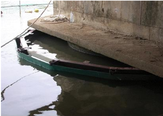
Coffer dam installation
