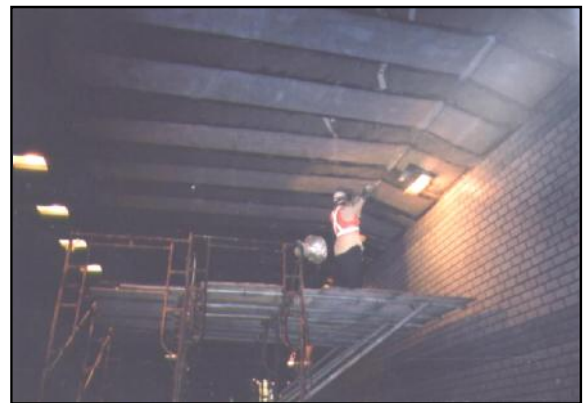
Adhesion of glass fiber
