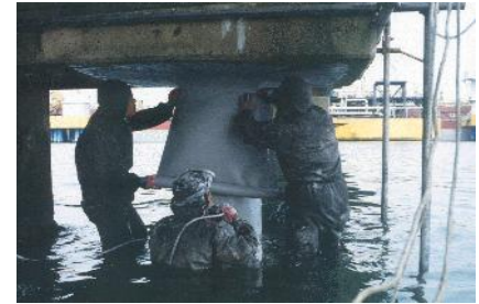
Ulsan SK 3 pier (under construction)
