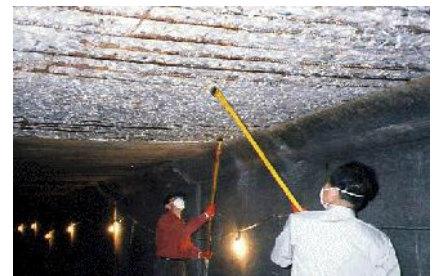
Old & new concrete paste
