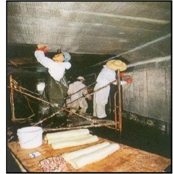
Adhesion of glass fiber
