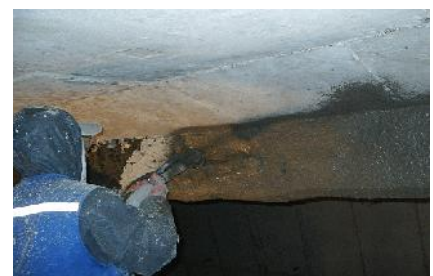
Rapid hardening cement spray
