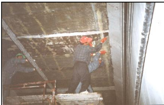
Adhesion of glass fiber
