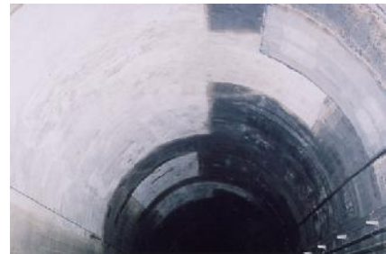
CAF application, Jinpyeong tunnel
