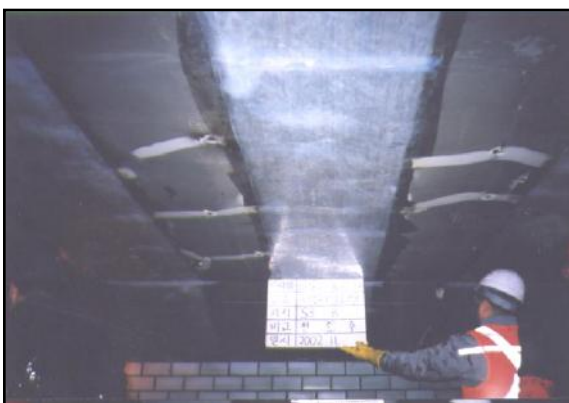
Adhesion of glass fiber
