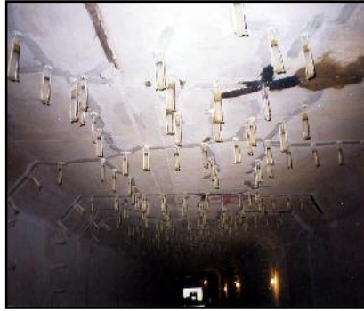
Crack repair (Epoxy injection)
