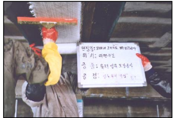
Adhesion of glass fiber
