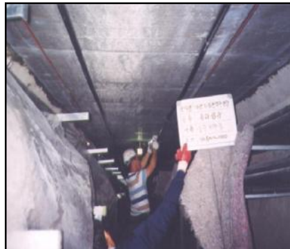
Adhesion of glass fiber
