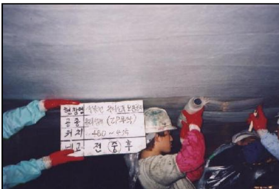
Adhesion of glass fiber
