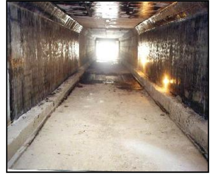
After Glass Fiber Reinforce
