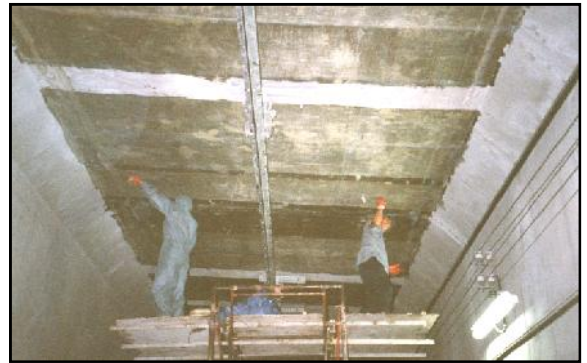
Adhesion of glass fiber
