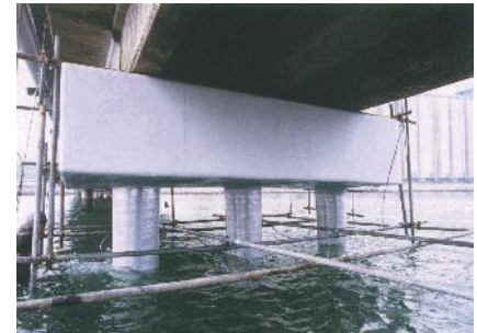
Ulsan SK 3 pier (after repair)
