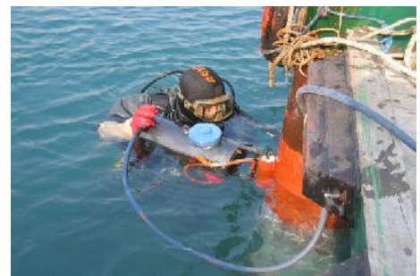
CAUW-COAT coating on steel
