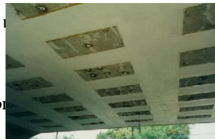
CAF application, Gungpyeong bridge
