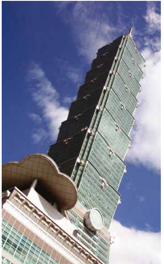
ABOVE: Taipei Financial Centre, Taipei, Taiwan. Also known as Taipei 101, this 508-metre structure makes a striking addition to Taipei's city skyline. Monokote® MK-6®/HY® and Z-146 were sprayed onto the structural beams and columns, and columns of the high-speed elevator shafts of this landmark project.
