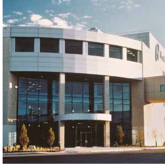
National Semiconductor Facility, South Portland, Maine, USA
